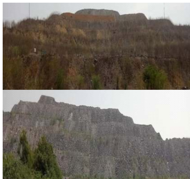
Fig. 2 (a & b): A typical view of the Waste Dump
